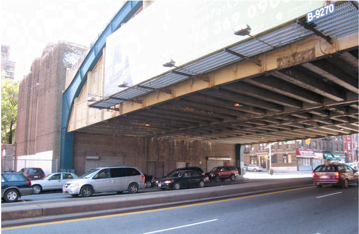
EXISTING CONDITION: 4 TH AVENUE, TOWARD EAST SIDE
