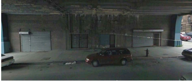
Current state of the decommissioned east side entrance
