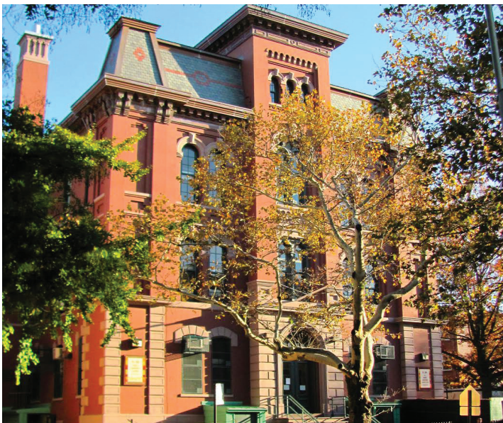
Restoration of PS 39 included reconstructing the school's slate tiled mansard roof, fabricating decorative copper work and restoring the original stone masonry.
