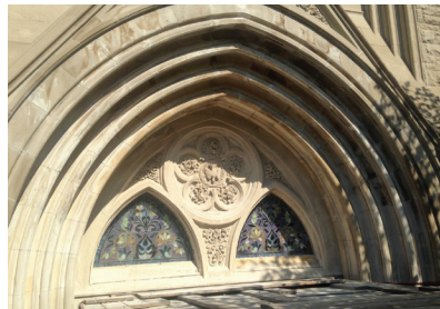
photo by Jan Hird Pokorny Associates
